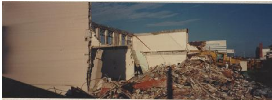
One of the Mid-Century Modern classroom building being demolished in 1994.
